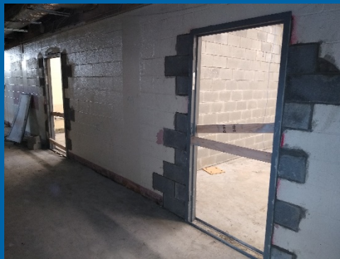
Installation of Door Frames in Masonry Walls
