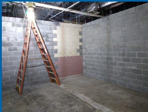
Top Out of Masonry Walls
