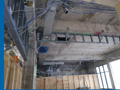
Install Drywall Framing at Entry
